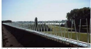
so as to be very flexible and spring back in their original position. From heights of 2 to 3 meters they can scarcely be seen, by which a building is not marred and absolutely protected from unwanted pigeons.
