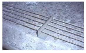
cm and a bar thickness of 1.3 mm. The width of this system varies according to the surface to be treated and the situation on the site. The length is endless because the bars are connected to each other by stainless steel springs.
