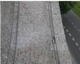
Because the cable is fully synthetic it allows mounting in any form which makes it also applicable on, for instance, monuments.
