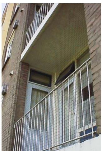
photo at an angle the net becomes visible. The edge finishing is realized by way of spanning stainless steel cables through stainless steel eyes placed and tensioned in advance by stainless steel spanners. After that the net is ringed onto the net mesh by mesh using stainless steel rings.
