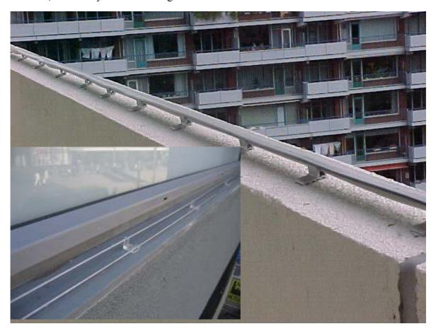
Above you see a practical application of the T-cable system on a concrete balustrade. This system is exclusively applied in those cases where extensive lengths are to be protected from birds and only in persistent cases. By using durable materials the life span is unprecedented and in case of maintenance of the base, the system can be easily dismounted temporarily and/or locally. For every practical application the system can be adapted to the desires of the customer.
